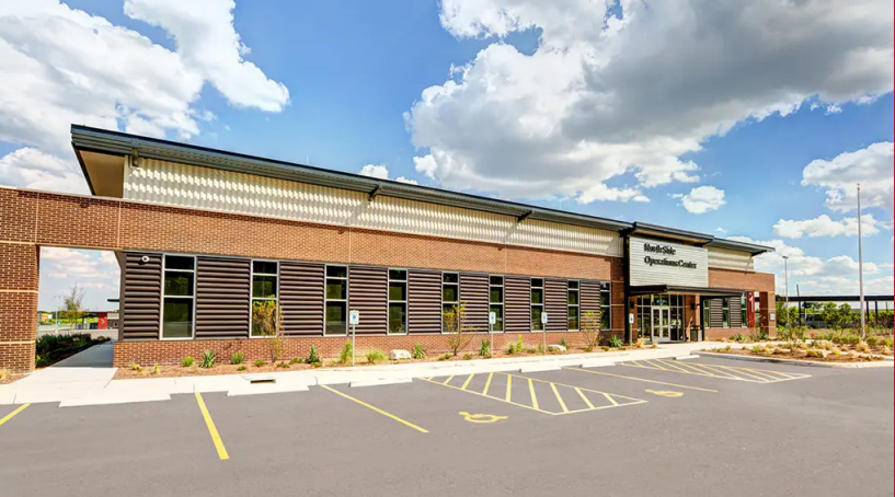
San Antonio Waste Water System New Operations Center - Design Build with DBR Engineering
