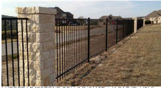
LEUDER LIMESTONE COLUMNS WITH 4" CAP (FLUSH)
