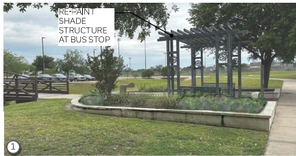
RE-PAIN SHADE STRUCTURE AT BUS STOP REMOVE ALL PLANT MATERIAL WITHIN 2FT FROM THE EDGE OF THE PLANTER, WATER-PROOF (LIQUID APPLICATION) BELOW COPING ALL THE WAY TO THE FOOTING OF PLANTER, SEAL AND RE-PLANT PLANTERS.
