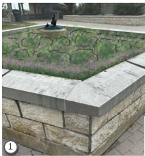
REFACE + RECAP + RE-PLANT PLANTERS. RESET CAP WITH SKATE STOPS
