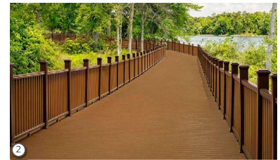
UPDATE BRIDGE SURFACE WITH TREX DECKING
