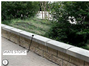
REFACE + RECAP + RE-PLANT PLANTERS. RESET CAP WITH SKATE STOPS
