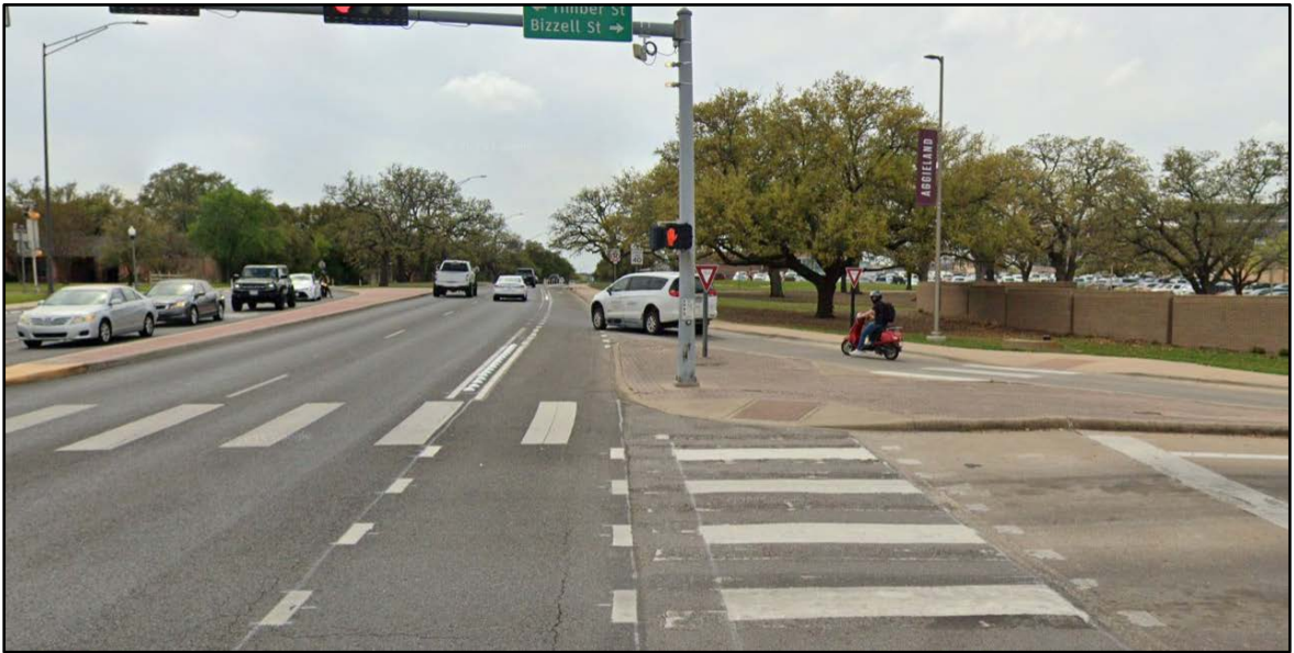
Slip lane for right turns to and from Bizzell Street create hazards for bicyclists and pedestrians
