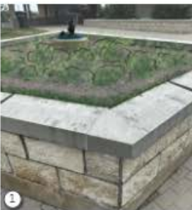
1 REFACE + RECAP + RE-PLANT PLANTERS. RESET CAP WITH SKATE STOPS
