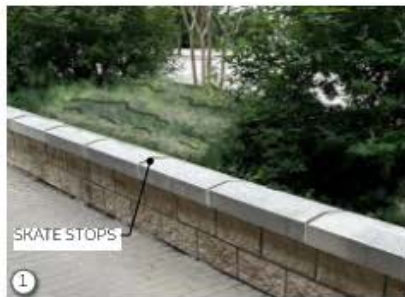
1 REFACE + RECAP + RE-PLANT PLANTERS. RESET CAP WITH SKATE STOPS
