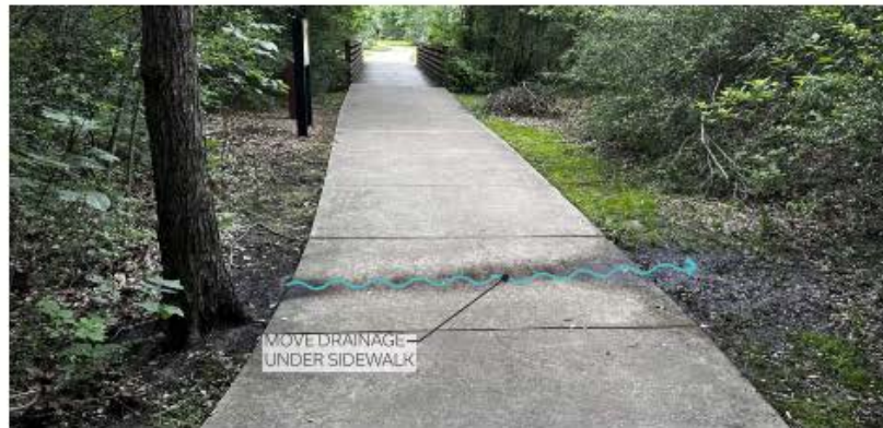
BORE AND ADD A PIPE UNDER SIDEWALK TO DAYLIGHT ON LOW SPOT OF ADJACENT LANDSCAPE AREA
