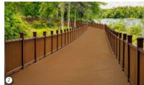
2 UPDATE BRIDGE SURFACE WITH TREX DECKING
