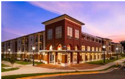
The Heritage at Cajun Village Lafayette, Louisiana
