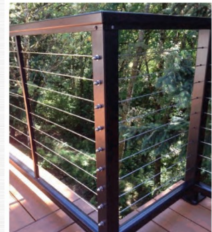
Cable rails/fencing painted black with stainless steel cables
