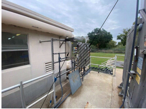
SCREENING FACILITY DEMOLITION PHOTO 1 PHOTOGRAPH A EH-1
