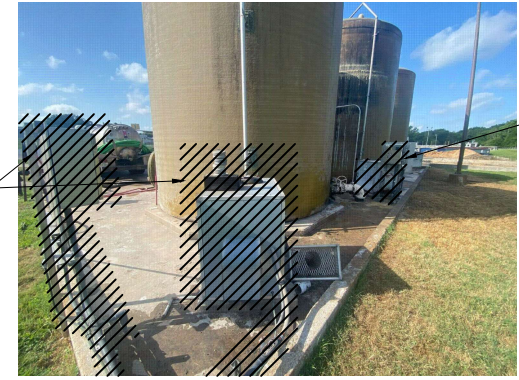
GREASE FACILITY DEMOLITION PHOTOGRAPH C NTS (10-DE-02)
