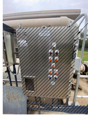
SCREENING FACILITY DEMOLITION PHOTO 2 PHOTOGRAPH B EH-1
