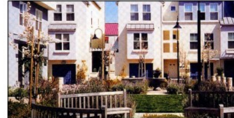
Town Houses or Row Houses 15 to 25 du/acre, 2 to 3 stories Surface parking or parking within each unit Source: Leland Consulting Group
