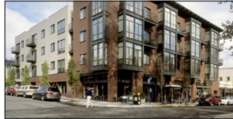
Wood Frame Condos or Apartments 20 to 35 du/acre, 2 to 3 stories Surface, garage or tuck under parking Source: Leland Consulting Group
