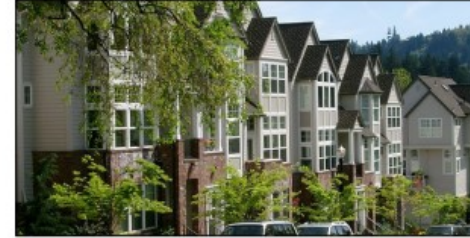
Mixed Use Mid-Rise 40 to 60 du/acre, 4 to 6 stories Structured parking Source: Leland Consulting Group
