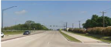
4 TEXAS AVENUE RAISED MEDIANS
