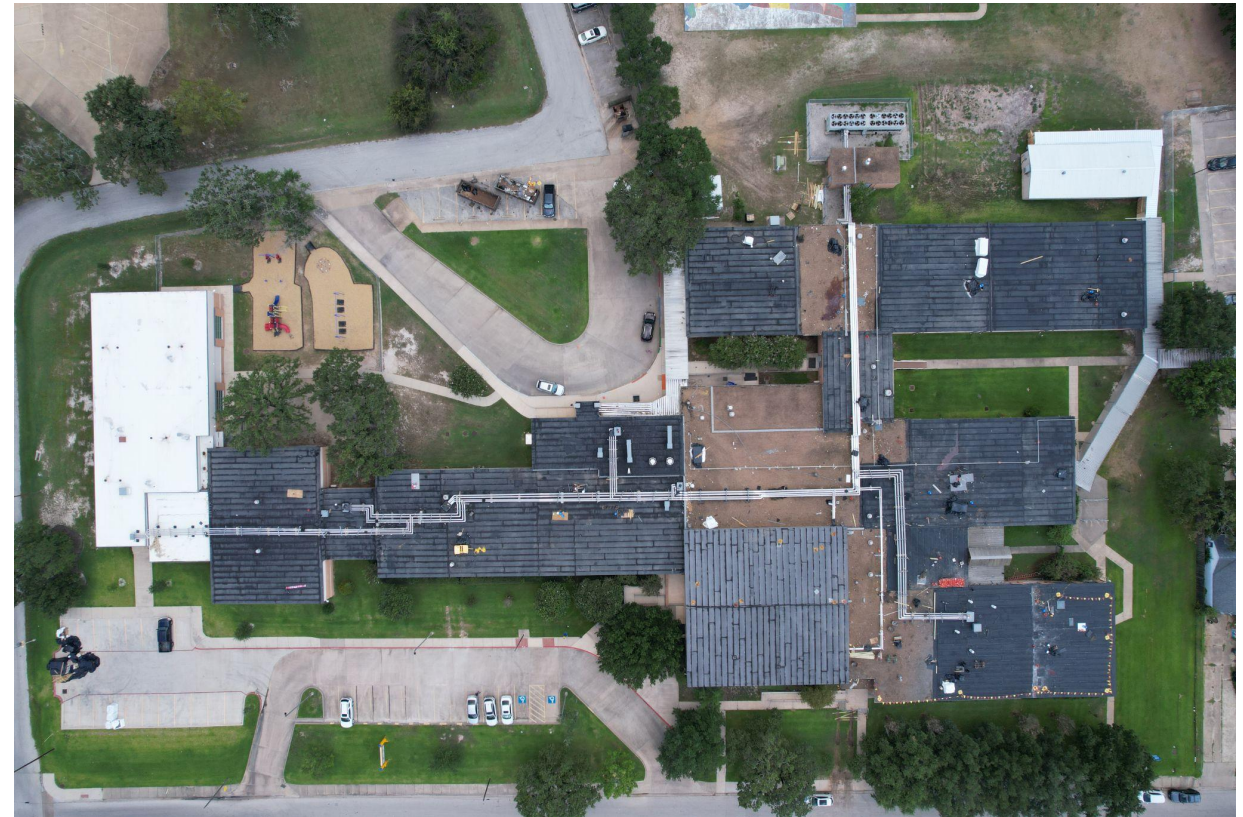
Crockett Elementary School Roof
