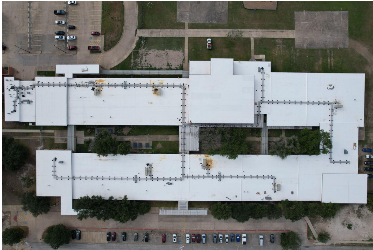
Jones Elementary School Roof
