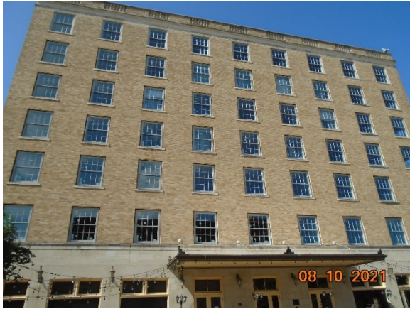
New windows in place in all guest rooms
