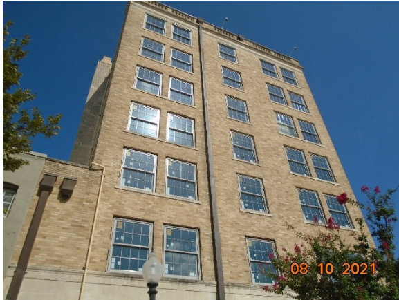
New windows – West side
