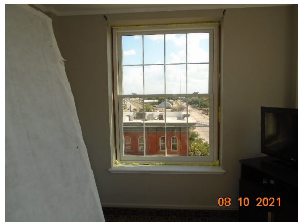
View of window in place, trimming in progress
