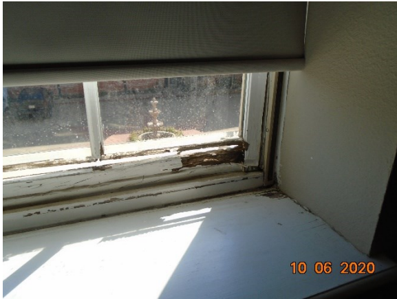
Old damaged windows have been removed.
