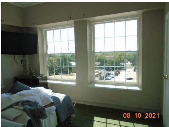
Interior view of 7 th floor new windows trimmed
