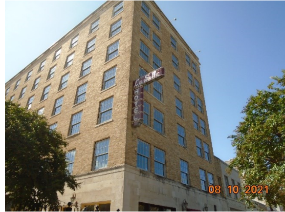
New windows in place – courtyard and East side
