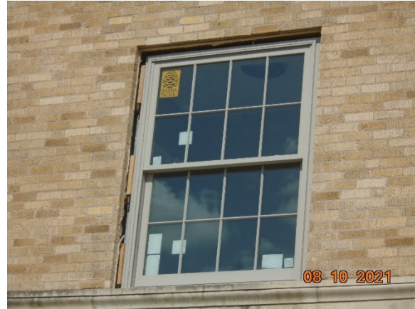
Close up of new windows.
