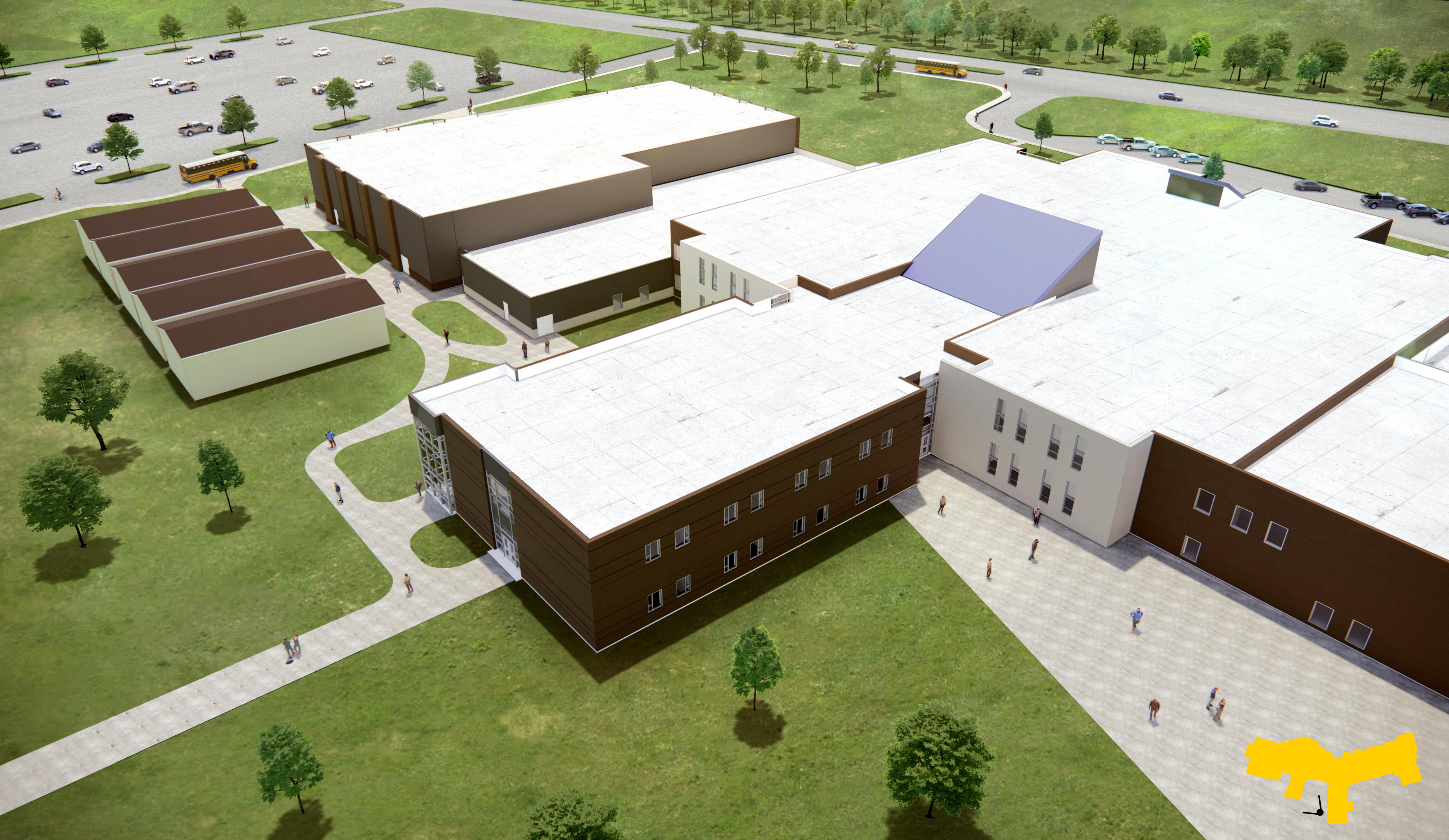
RUDDER HIGH SCHOOL - EXTERIOR VIEW 01
