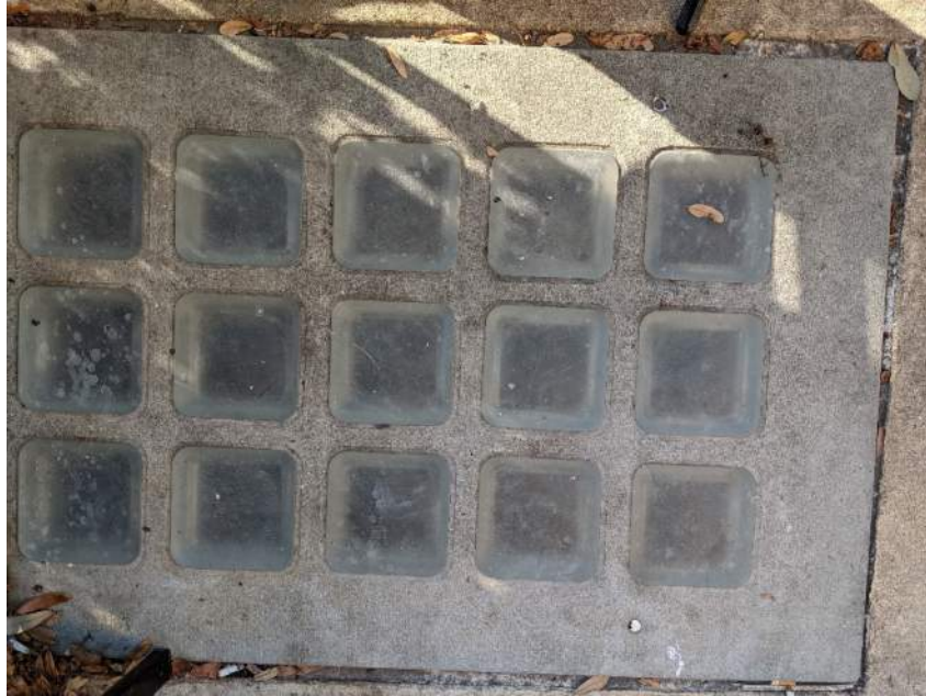
Figure 8 - Sidewalk Windows from Above
