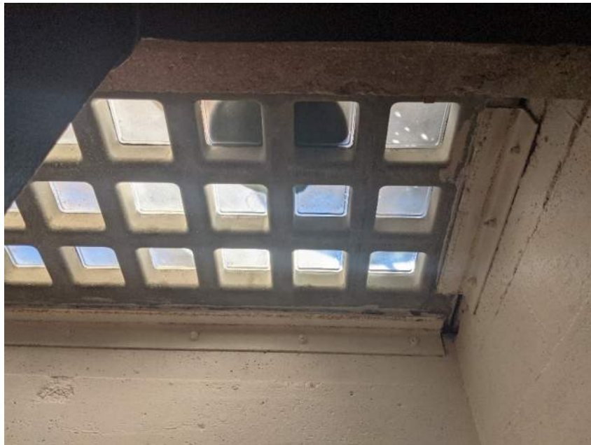
Figure 9 - Sidewalk Windows from Below
