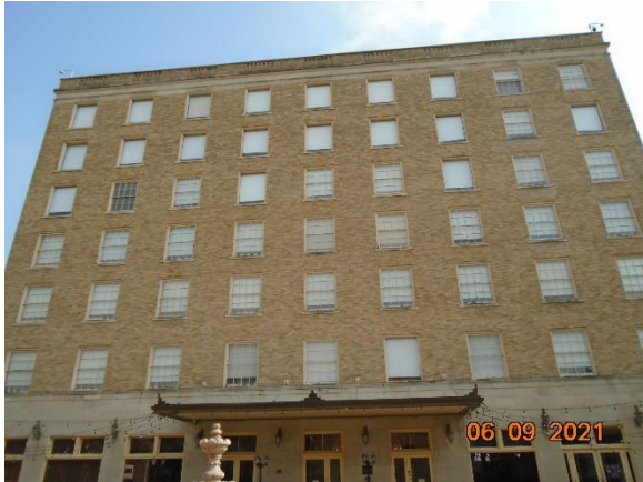
More wood sashes removed on South side
