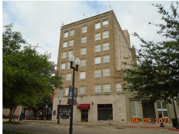
More wood sashes removed on East Side
