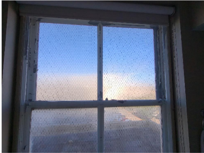
Top of steel framed window:
