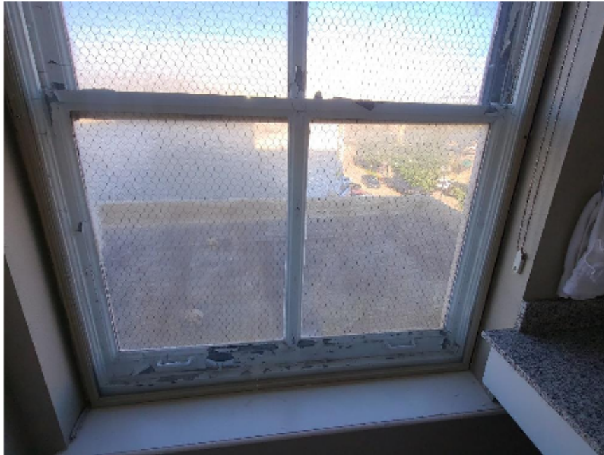
Bottom of Steel framed window:
