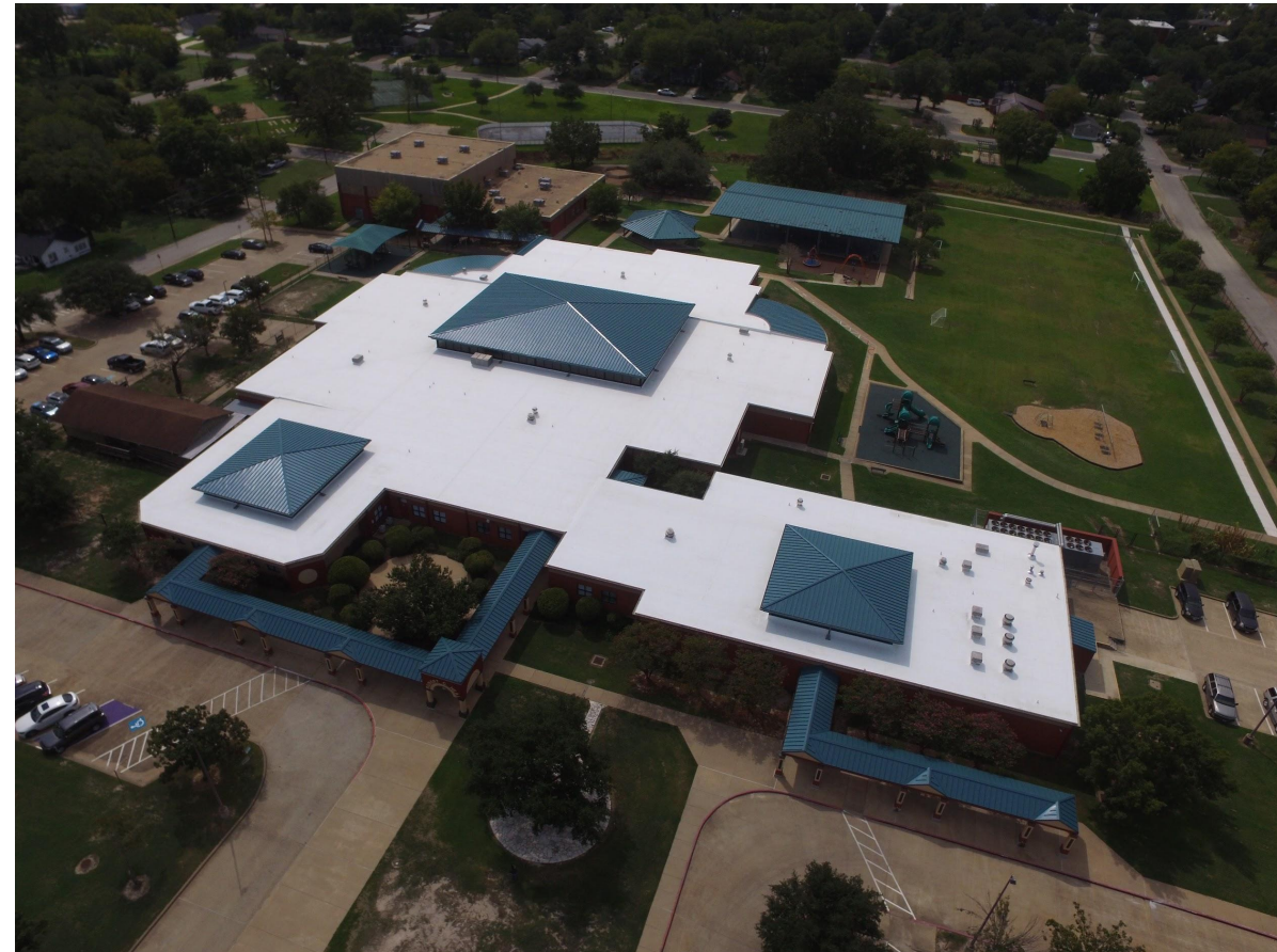
Neal Elementary Roof Replacement
