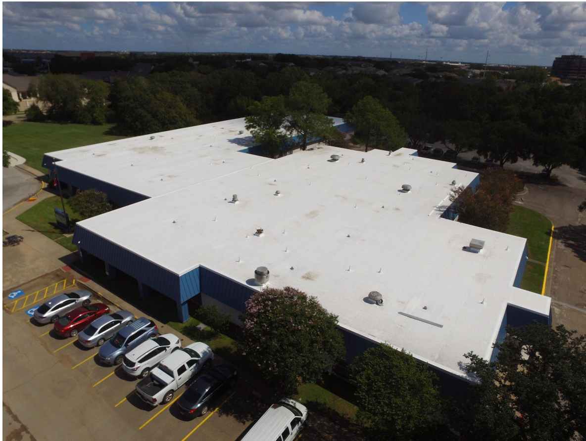
MC Harris Roof Replacement
