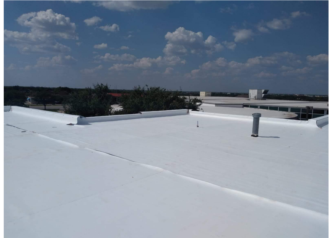
Bryan High School Roof Replacement
