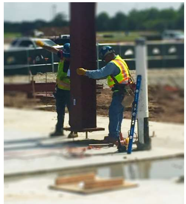
IRON WORKERS PLACE THE FIRST STRUCTURAL STEEL
