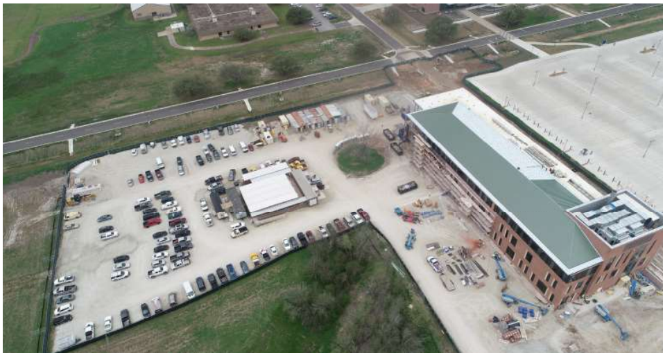
AN AERIAL VIEW DURING CONSTRUCTION
