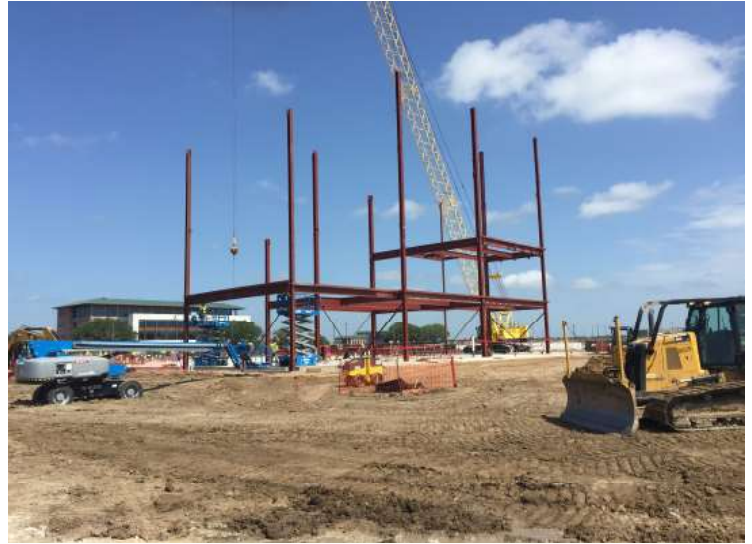
THE BUILDING BEGINS TO TAKE SHAPE AND THE SITE IS PREPARED
