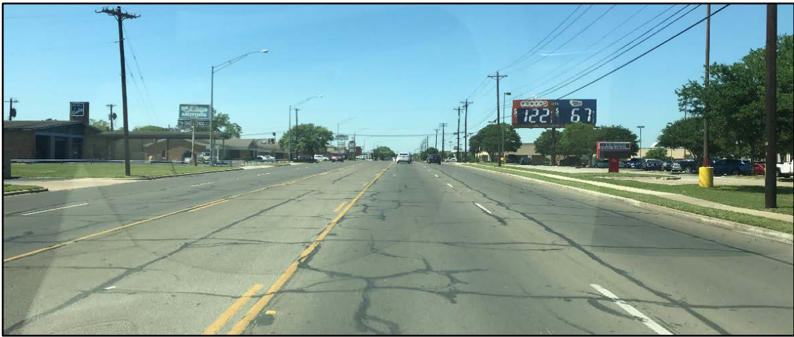
Figure 5 – Northbound S. Texas Ave. in front of HSA (View looking north)
