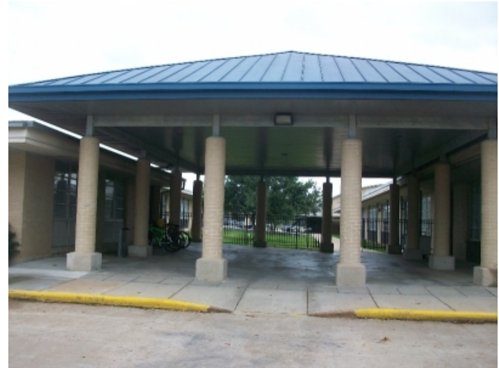
EXISTING BUILDING ENTRIES
