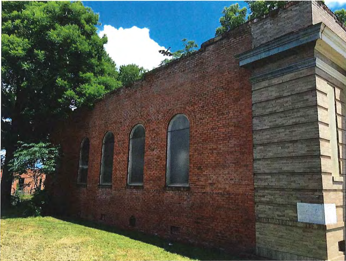
North wall, view facing southeast
