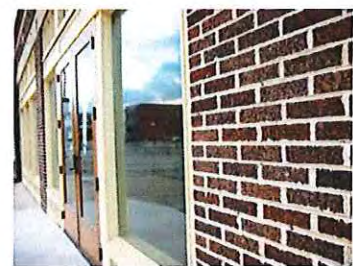
308 N. Bryan Ave. Downtown Bryan, Texas A seventy-year-old dry goods store turned into offices for a cutting-edge architecture firm.
