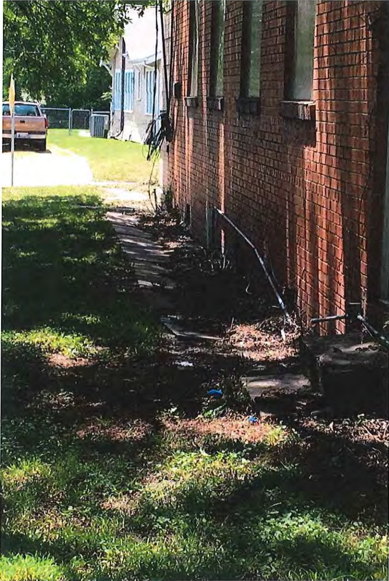
Detail – south wall, view towards west, ground slopes toward building
