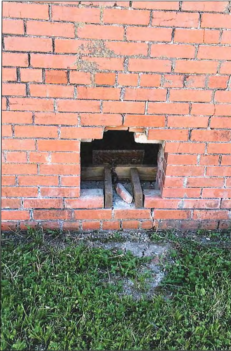
Detail – crawlspace vent, north wall
