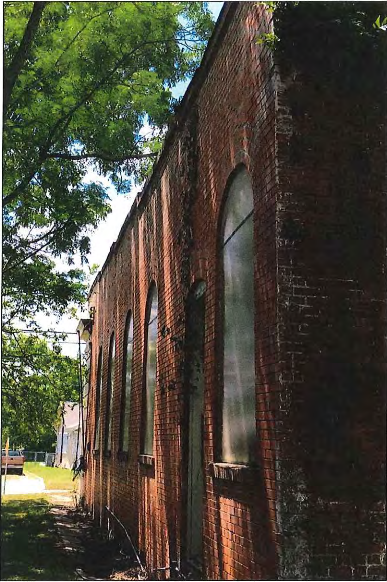
View along south wall facing west
