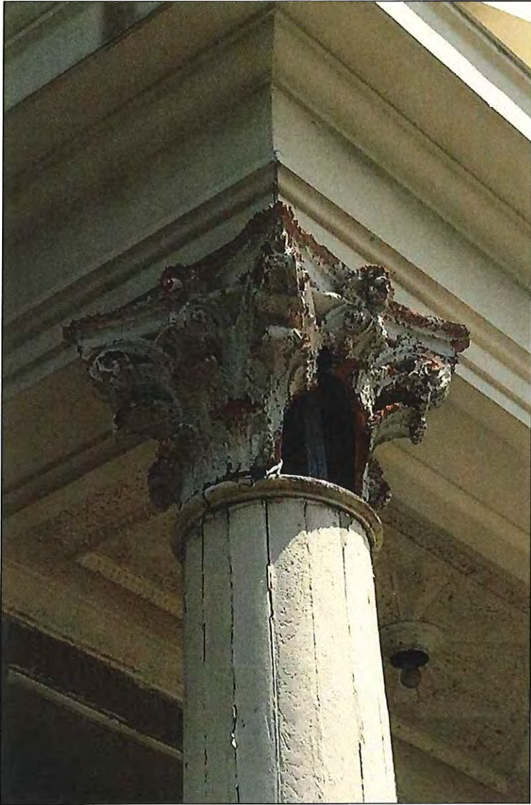
Detail - column capital
