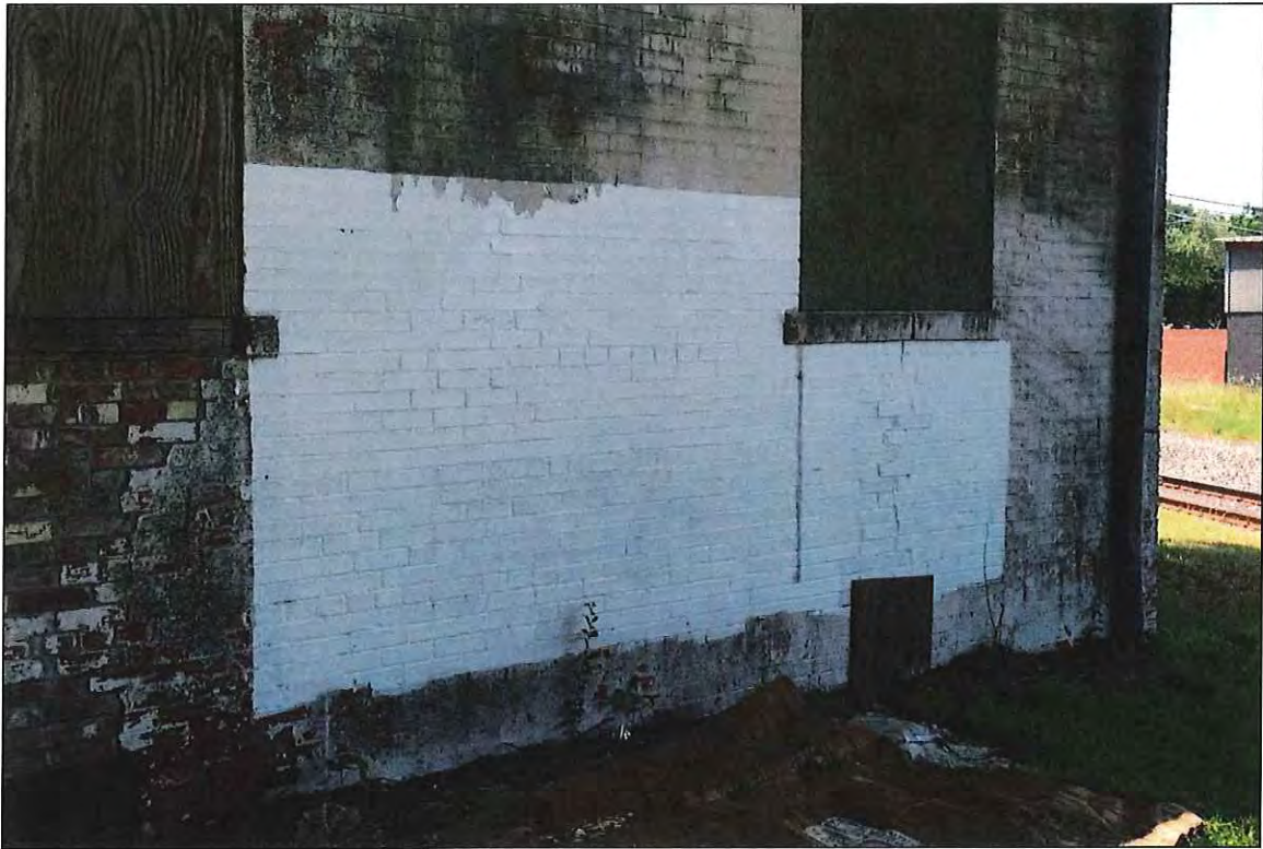
Lower portion Rear (east) wall, view facing northwest
