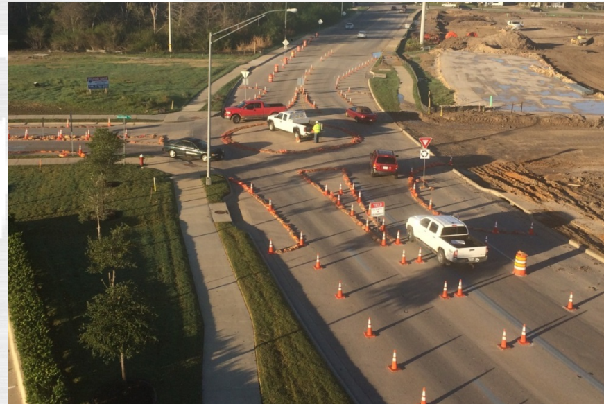
Temporary testing of a mini roundabout at Broadmoor Drive and Nash Street
