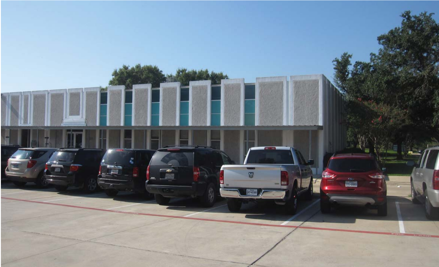
EXISTING DINING FACADE
