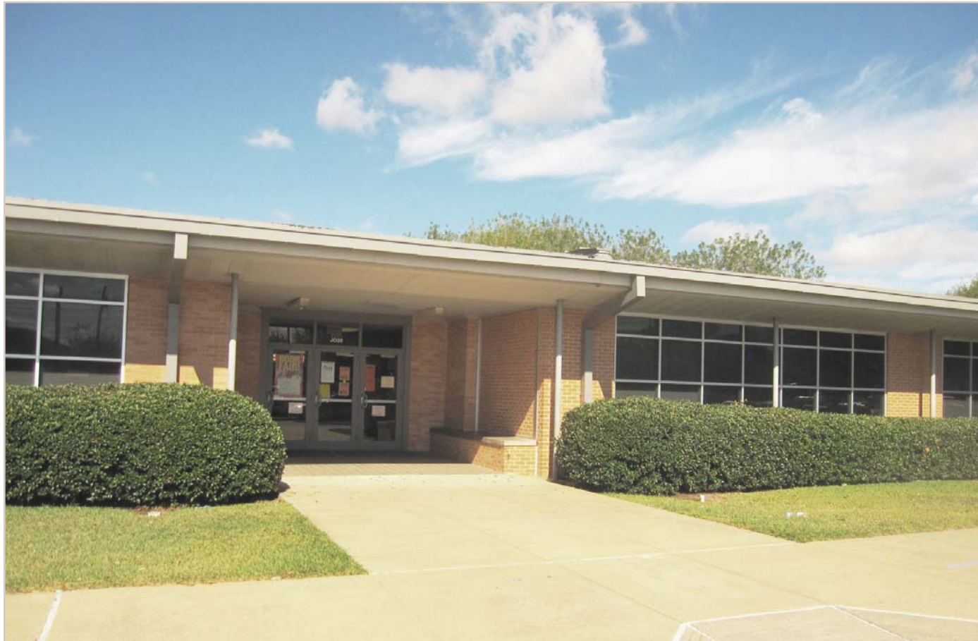
EXISTING DROP OFF ENTRANCE
